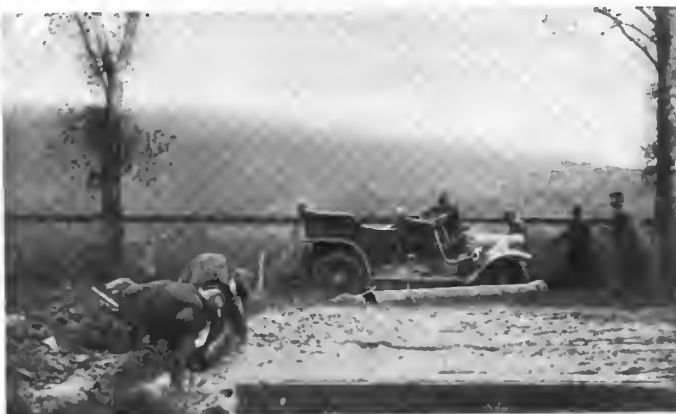
WHITE TACKLES A BERKSHIRE ROAD IN PROCESS OF REPAIR.
